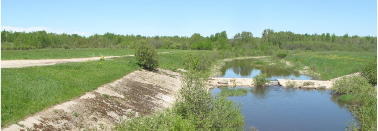
Bennett – West Davignon Diversion Channel – Base Line Rd
