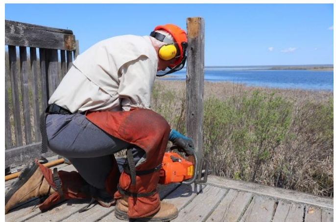
2019 removing upper deck railing
