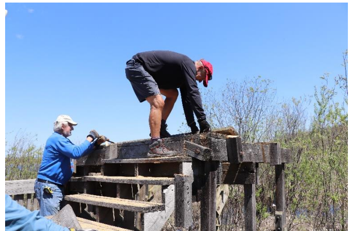
2019 upper deck removal
