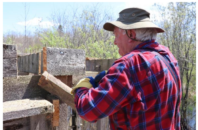
2019 upper deck removal
