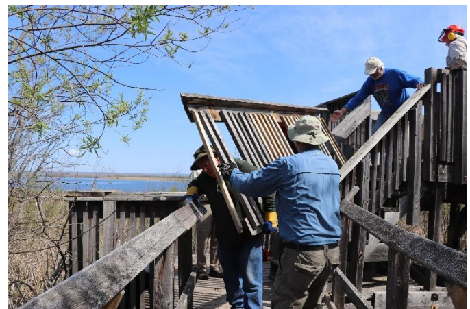
2019 removing upper deck railing
