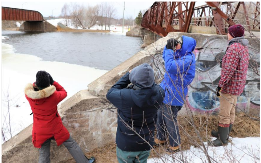
Old train bridge in Echo Bay - Val Walker
